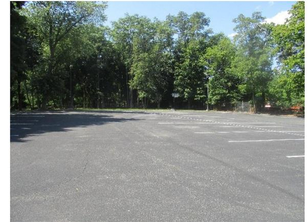
Parking spots west of the building can be replaced with porous asphalt to capture and infiltrate stormwater runoff. A preliminary soil assessment suggests that the soils have suitable drainage characteristics for green infrastructure.
