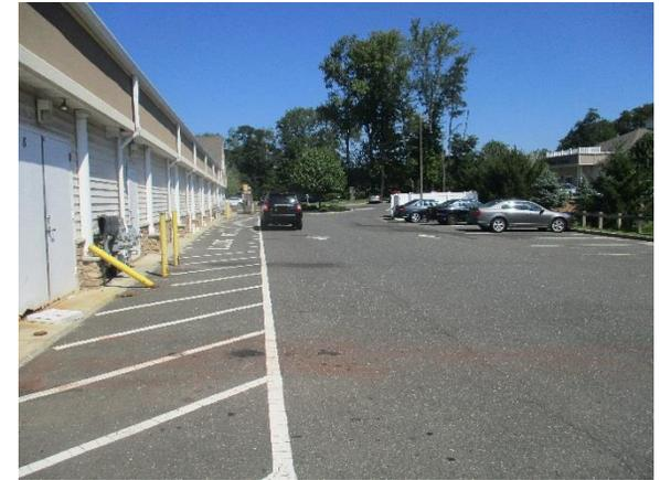
Parking spaces can be replaced with porous asphalt to capture and infiltrate runoff. A preliminary soil assessment suggests that the soils have suitable drainage characteristics for green infrastructure.
