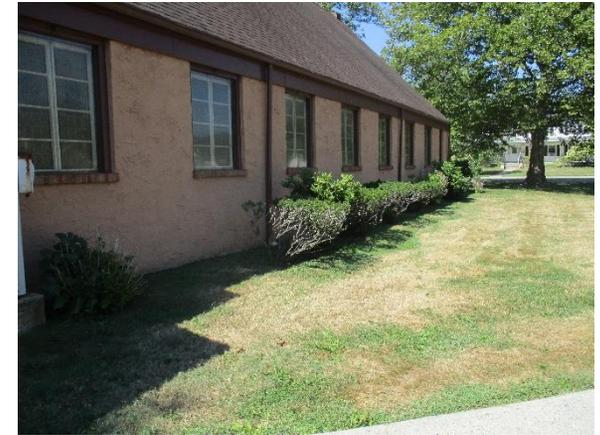
Parking spaces can be replaced with porous asphalt to capture and infiltrate stormwater. Installing rain gardens adjacent to the building can capture, treat, infiltrate roof runoff. A preliminary soil assessment suggests that the soils have suitable drainage characteristics for green infrastructure.
